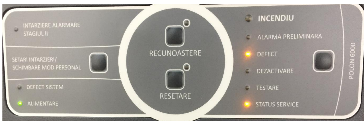
Figure 6.3/1 User interface - keyboard + signalling devices
