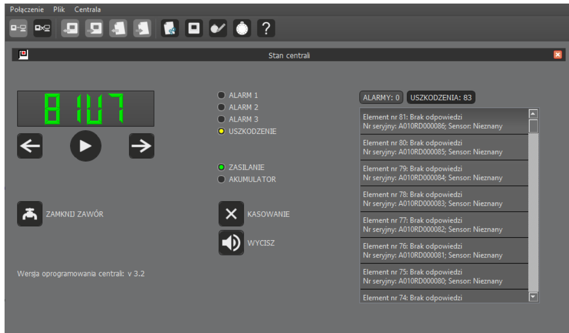
Figure 4.4/1 Tab displaying the control panel status
